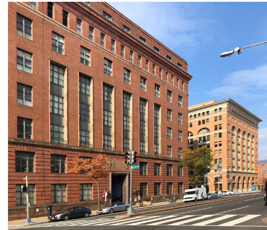
Government Printing Building (South of Site)
