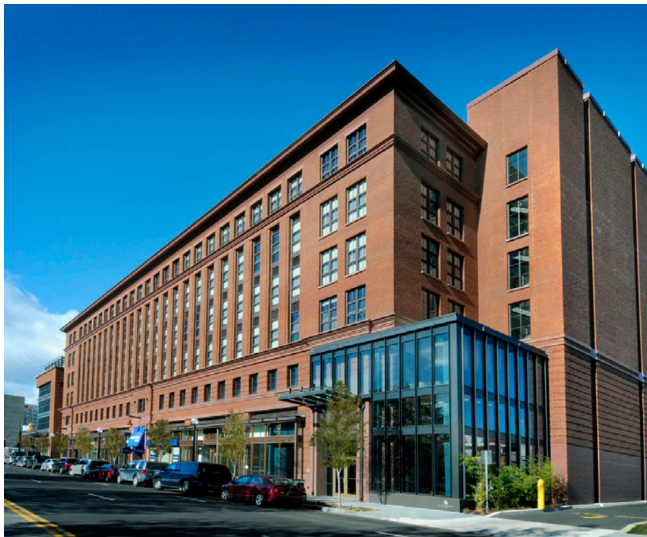
77 H Street (West of Site)
